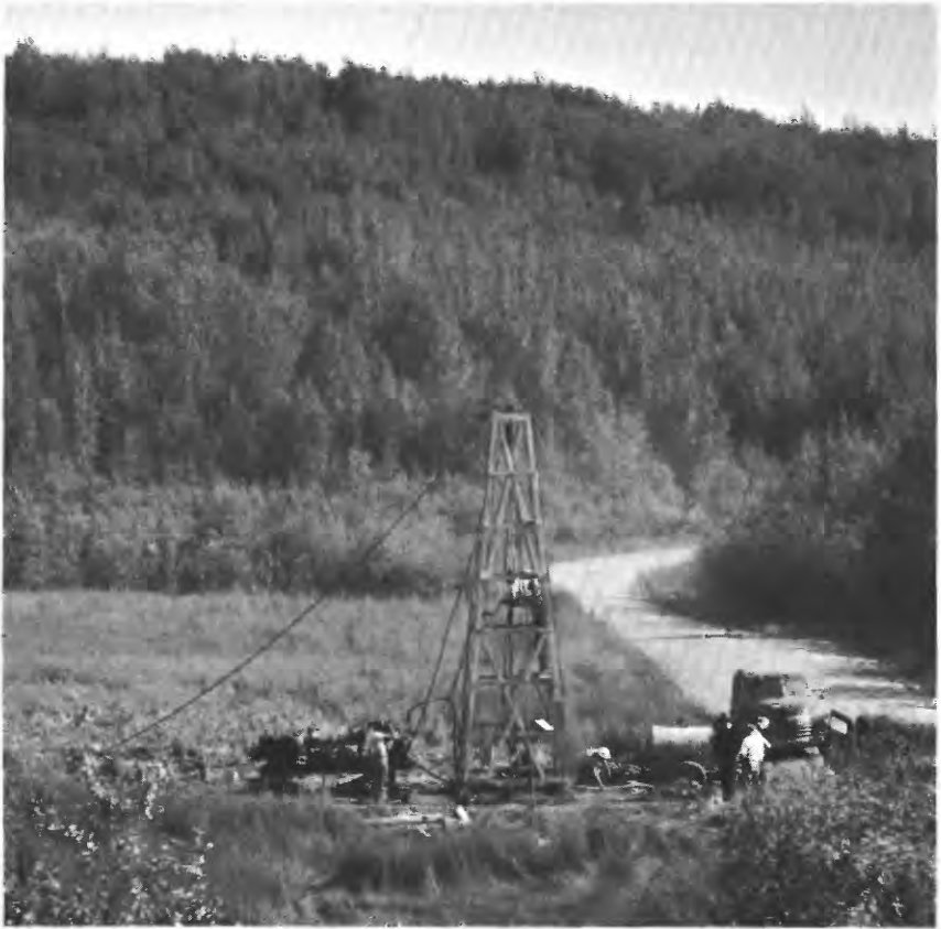
FIGURE 7.—Experimental jet drill used in 1954. Test hole being drilled in subordinate valley in low mountains north of Fairbanks.
