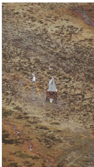
Weather Monitoring Station located near toe of proposed TSF
