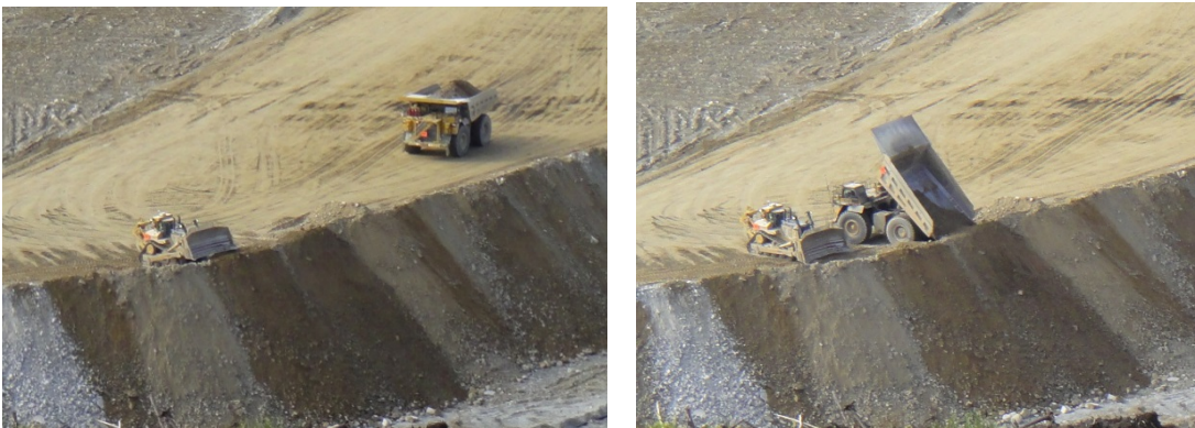
Figure 5-1: Typical Waste Rock Dump Construction
