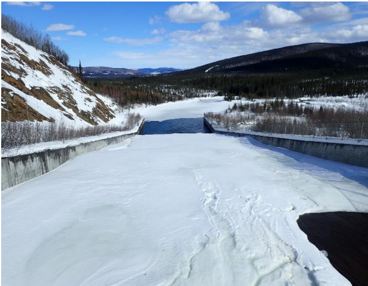
Figure 6. Spillway at outlet of Water Supply Reservoir on April 15, 2021.
