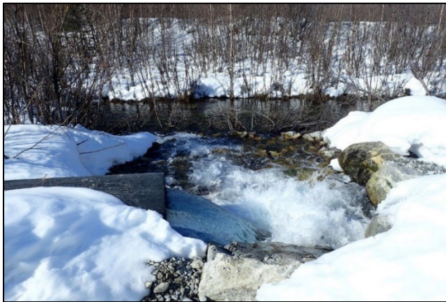
Figure 4. Outfall 002, RO water discharge of up to 3,000 gpm into the RO Channel Wetlands.
