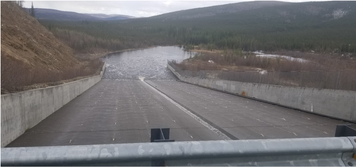
Figure 3. Spillway in water supply reservoir in late April 2018.
