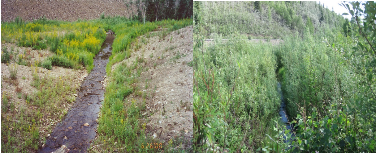
Figure 2. Pond F outlet channel in 2000 (left photo) and in 2010 (right photo).
