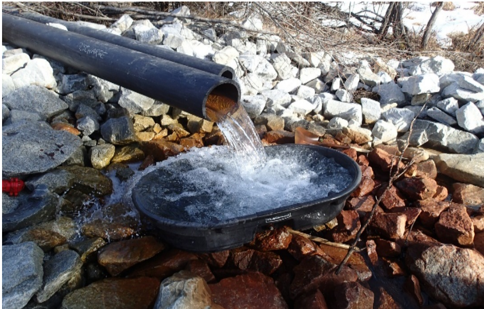
Figure 9. Discharge point for non-contact water from dewatering wells around the Fort Knox open pit.
