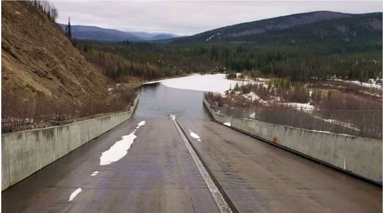
Figure 4. Spillway at outlet of water supply reservoir (WSR) on April 10, 2019.
