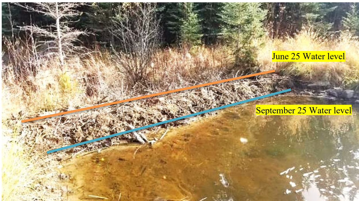
Figure 41. Comparison of Fort Knox Stilling basin water level, June and September 2019.
