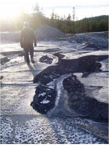
Tailings Disposal Site – Southeast Expansion Area 2 Note: Rill Erosion from previous precipitation events
