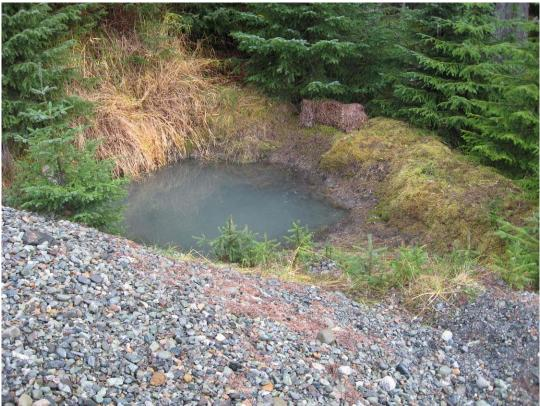
Photo 3. The settling basin leads to a second sediment catchment with a bale at the outlet.
