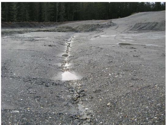
Photo 5. Bales will be placed in this drainage ditch to catch sediments.
