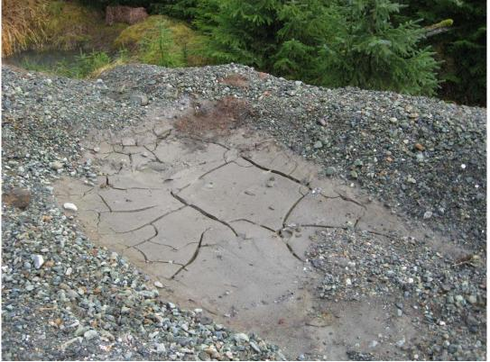
Photo 2. Drainage ditch leads to a settling basin.
