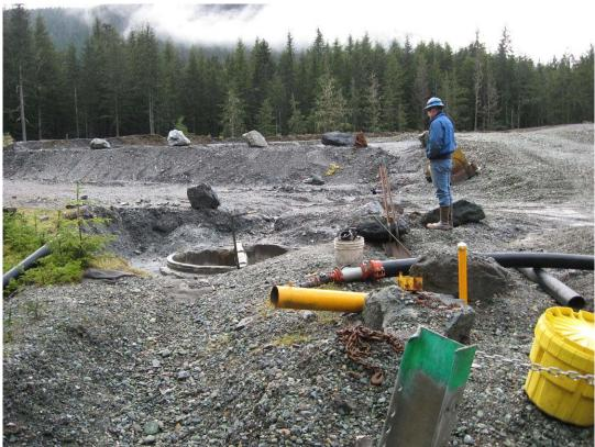
Photo 1. Pump sump at Site E and drainage ditch
