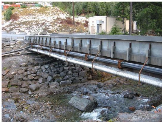
Photo 7. New double-walled pipes at the 920 bridge.
