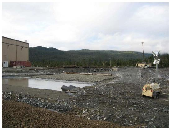
Photo 9. Pond 7 pre-sedimentation basin and pad for filter bags.
