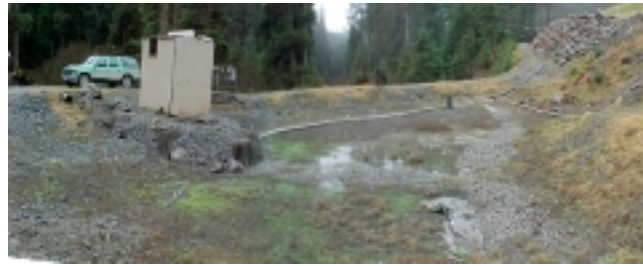
Site D Berm – Inside and pump house over wet well
