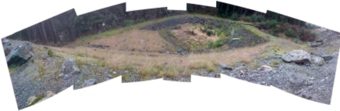
Site “C” Panorama of Downgradient Aspect – Note Proximity of Greens Creek
