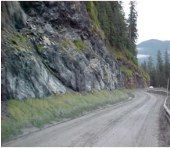
Blasted Rock Along Mi 2.5 B-Road
