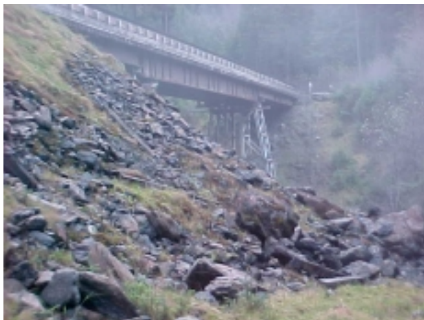
Zinc Creek Bridge Abutment
