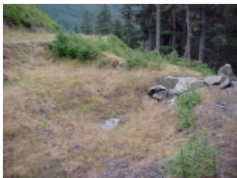
Old, breached Sediment Pond at Site 1350
