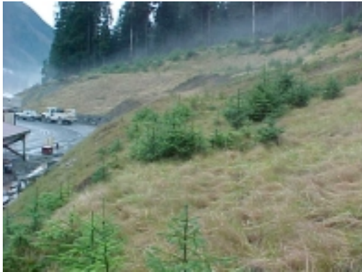
Site 920 Millsite Backslope
