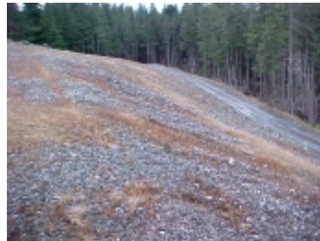
Waste Site E – Northwestern Aspect
