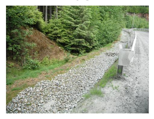
PHOTO 1. Ditch stabilization measures above 3.0-mile bridge.
