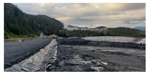
PHOTO 6. Capping tailings with waste rock to control erosion and fugitive dust.
