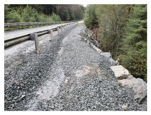
PHOTO 2. Stabilized slope and reconstructed ditch at 3.2-Mile.
