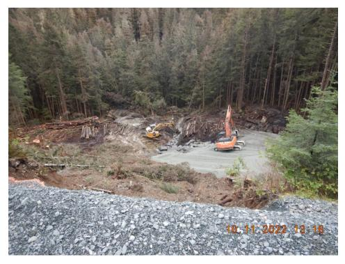
PHOTO 4. Preparing foundation for buttress below 5.6-Mile after landslide.
