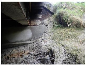
Photo 22. Sediment accumulation continues below Falls Creek Bridge.
