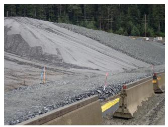
Photo 29. Class 1 waste rock was placed along sections of the outer slope.
