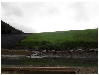
Photo 30. Hydroseeded northwest slopes in the TDF area.
