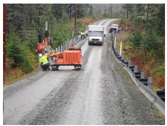
Photo 3. Contractors installing guardrails along the A-road.
