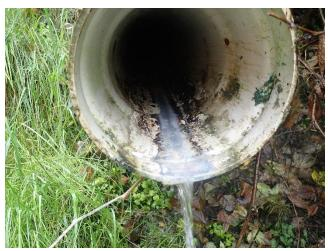
Photo 27. The cleaned abutment drain.
