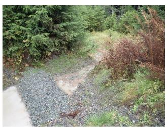
Photo 23. The final settling pond/rock check damn for the 3.2 mile B-road culvert.
