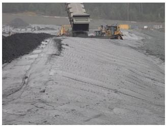
Photo 31. HGCMC continues placing tailings in the S3P1 area.
