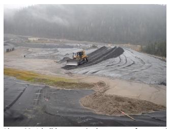
Photo 32. A bulldozer was in the process of compacting and contouring a tailings pile in the S3P1 area.
