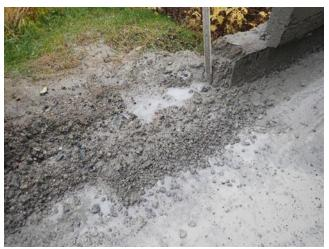
Photo 16. Sediment accumulation at the bridge ends for 3.4 mile B-road Bridge (Falls Creek Bridge).
