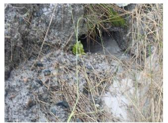
Photo 20. Sediment accumulation has exceed the allowable amount at the 3.4 mile B-road culverts intake.
