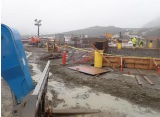
Photo 30. Contractors continue with the construction of the TDF wheel wash station.
