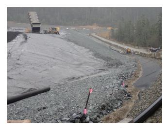
Photo 29. The rock placed at the toe of the tailings pile is from the 0.9 mile B-road rock stockpile.
