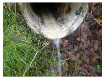
Photo 27. Zinc Creek abutment drain had mostly clear water flowing out.
