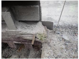
Photo 17. Sediment accumulation at the bridge end.
