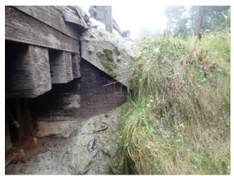
Photo 18. Some of the sediments have been removed. However, residual sediments still remain underneath the bridge.
