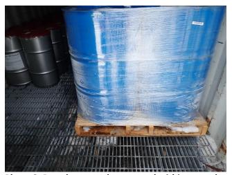
Photo 8. Petroleum products stored within secondary containment.
