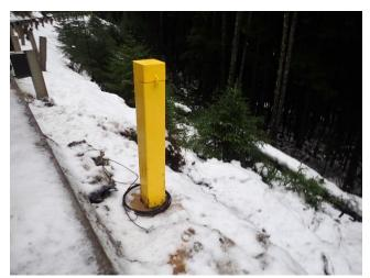
Photo 17. The inclinometers installed will be used for monitoring slope stability.
