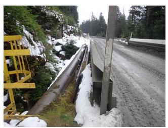
Photo 19. The splashguards are effectively working by preventing sediment splash over.
