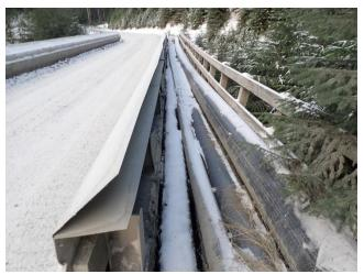
Photo 8. No sediments were observed on the pipeline.
