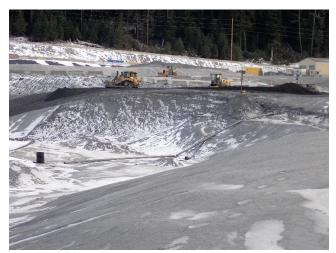
Photo 12. HGCMC continues placing tailings in the S3P1 expansion area.
