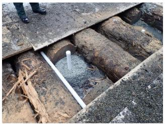
Photo 27. Two inclinometers installed at this location.
