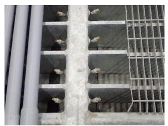
Photo 21. The water jets for the wheel washing station.
