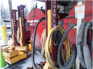
Photo 8. The maintenance shop's two 5,000-gallon tanks containing motor oil and hydraulic fluid.
