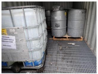
Photo 6. Storage containers in secondary containment.
