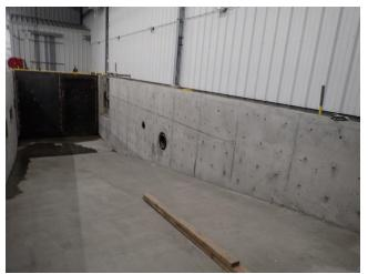
Photo 19. A de-grit basin inside the wheel wash station.
