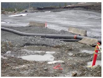
Figure 19. The wheel wash station drainpipe to Pond 7.
