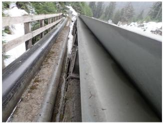
Photo 9. Splashguards are effectively working to prevent sediment splash over.
