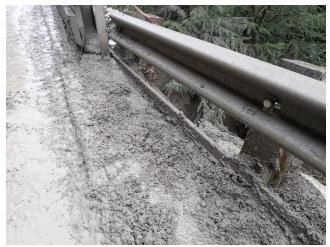
Photo 13. Sediment accumulation at the bridge end.
