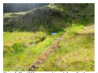
Photo 3. The 1350 pump and trench for collecting contact water from remnant waste rock piles.
