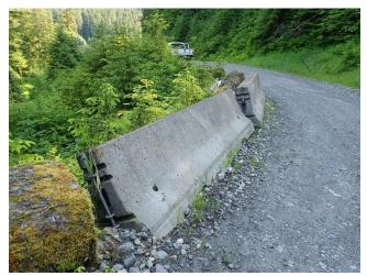
Photo 1. Now restaged, the jersey barrier that was leaning along the edge of the 1350 access road.
