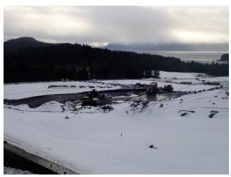
Photo 14. HGCMC is activiely placing tailing along the eastern ridge of the S3P1 area.
