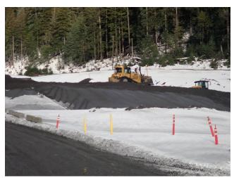
Photo 13. Tailings being desposited and compacted in the S3P1 area.
