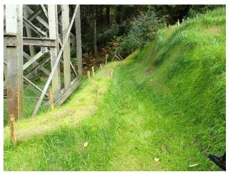
Photo 14. New compost wattles were placed and seeding undreneath the bridge.
