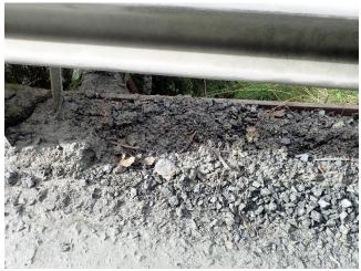
Photo 11. Sediment removal is required at the bridge ends.
