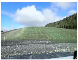
Photo 19. The southern section of the S3P1 area has been hydroseeded.
