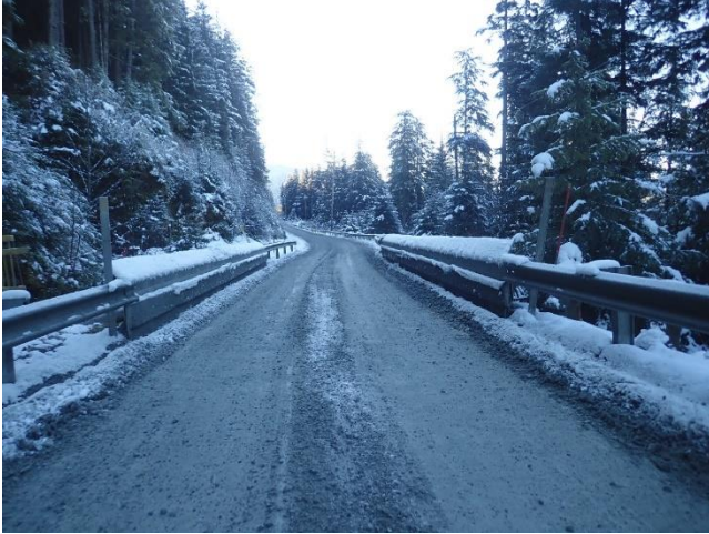
Photo 22. The 3.4 Mile B-road Bridge (Falls Creek Bridge).
