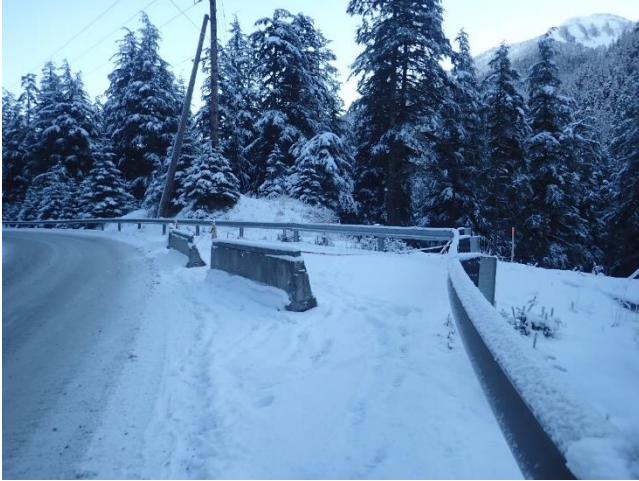
Photo 10. B-road adjacent to 7.5 mile landslide.
