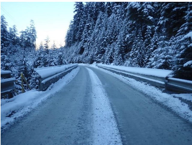
Photo 21. 7.4 Mile B Road Bridge (Killer Creek Bridge).
