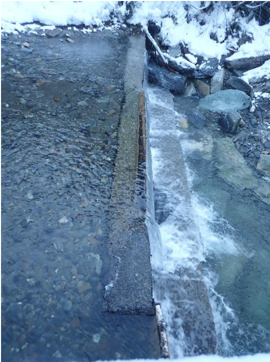
Photo 3. The 920 Greens Creek weir.
