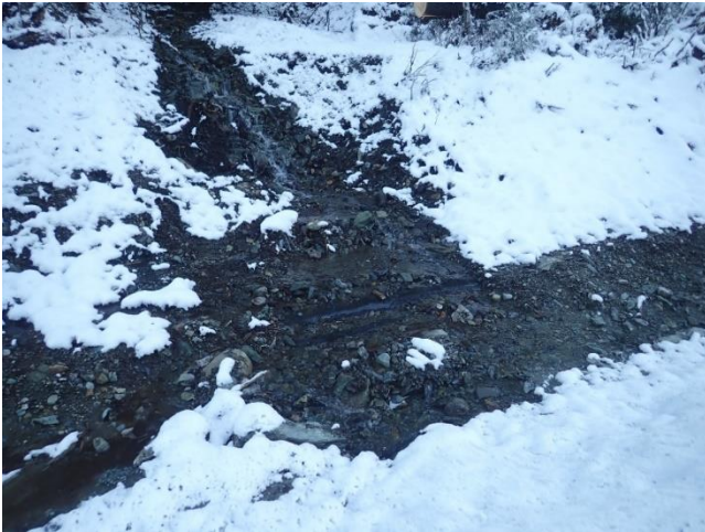
Photo 17. Site of 3.7 mile B-road landslide from December storm.
