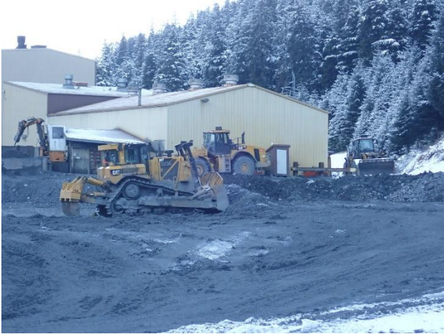
Photo 1. 920 ore pad and mill exterior.
