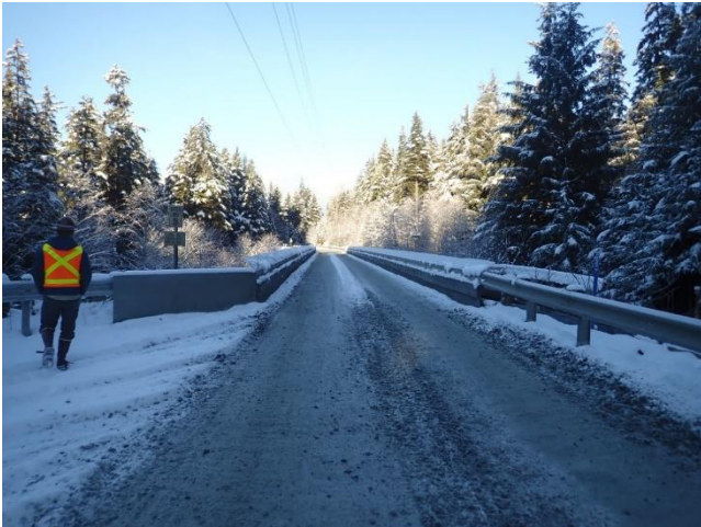
Photo 23. The 3.0 mile B-road bridge (Zinc Creek bridge).
