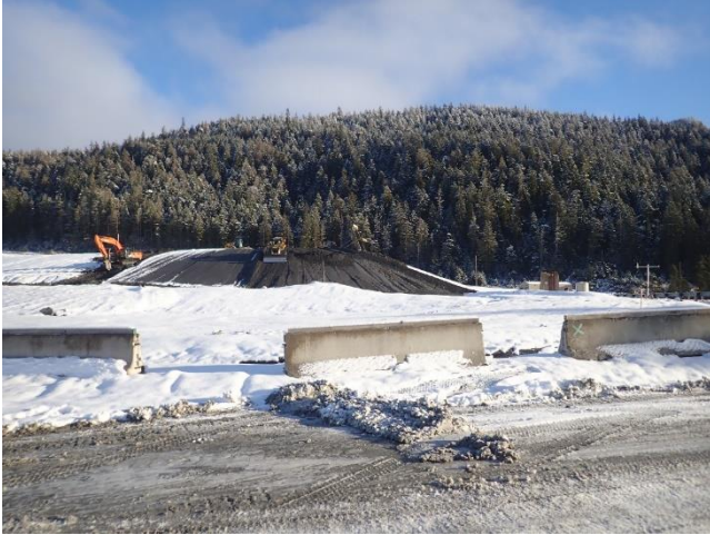
Photo 28. TDF S3P1 area. Personnel were actively placing tailings during the inspection.
