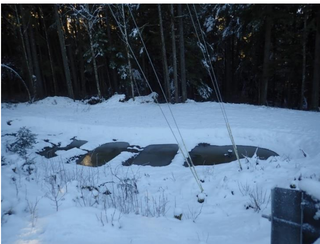
Photo 24. 3.0 mile B-road uphill abutment BMP's.
