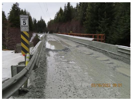
Photo 15. Surface of Zinc Creek Bridge showing ponding at bridge end.
