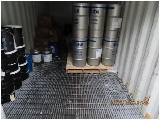
Photo 6. Chemicals in appropriate secondary containment at the 920 area warehouse.
