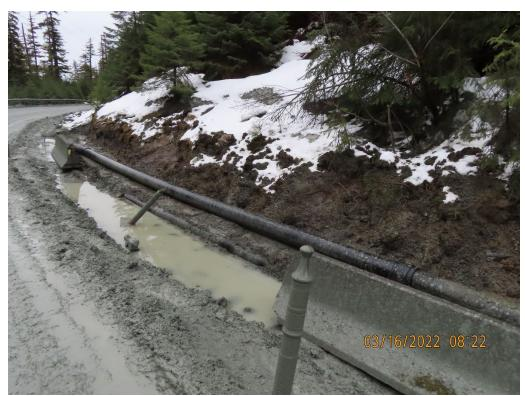
Photo 1. Repaired section of 10" HDPE pipe at approximately 5.1-mile B-Road.
