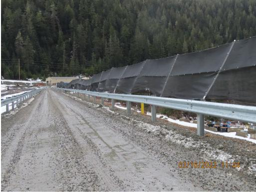
Photo 20. Damaged fugitive dust fencing south of the TDF.
