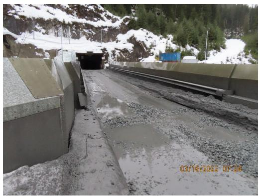
Photo 5. Greens Creek Mine portal and 920 bridge, showing functioning splash guards.
