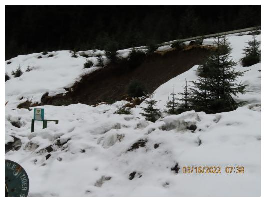
Photo 7. New slump observed below access road north of the warehouse area.
