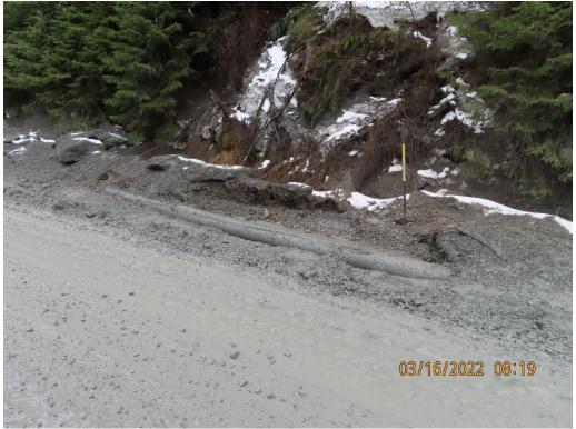
Photo 2. Damaged section of 8" HDPE pipe at approximately 5.7-mile B-Road.
