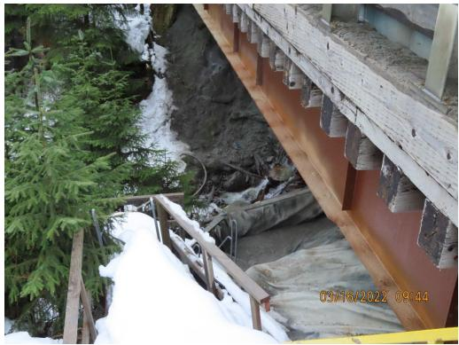
Photo 11. Killer Creek Bridge downhill side abutment showing BMPs in disrepair.
