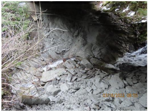
Photo 13. Below Falls Creek Bridge, showing excessive sediment accumulation without BMPs to prevent impacting surface waters with sedimentation and/or turbidity.
