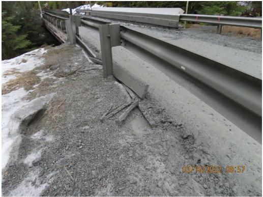
Photo 14. Damaged sediment deflection boards at Falls Creek Bridge.
