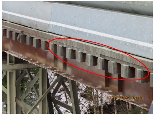
Photo 16. Closeup of turbid water overtopping bridge liner at Zinc Creek Bridge. Photo was taken immediately following the passage of a Max Haul truck, which produced the water in this photo, circled in red.
