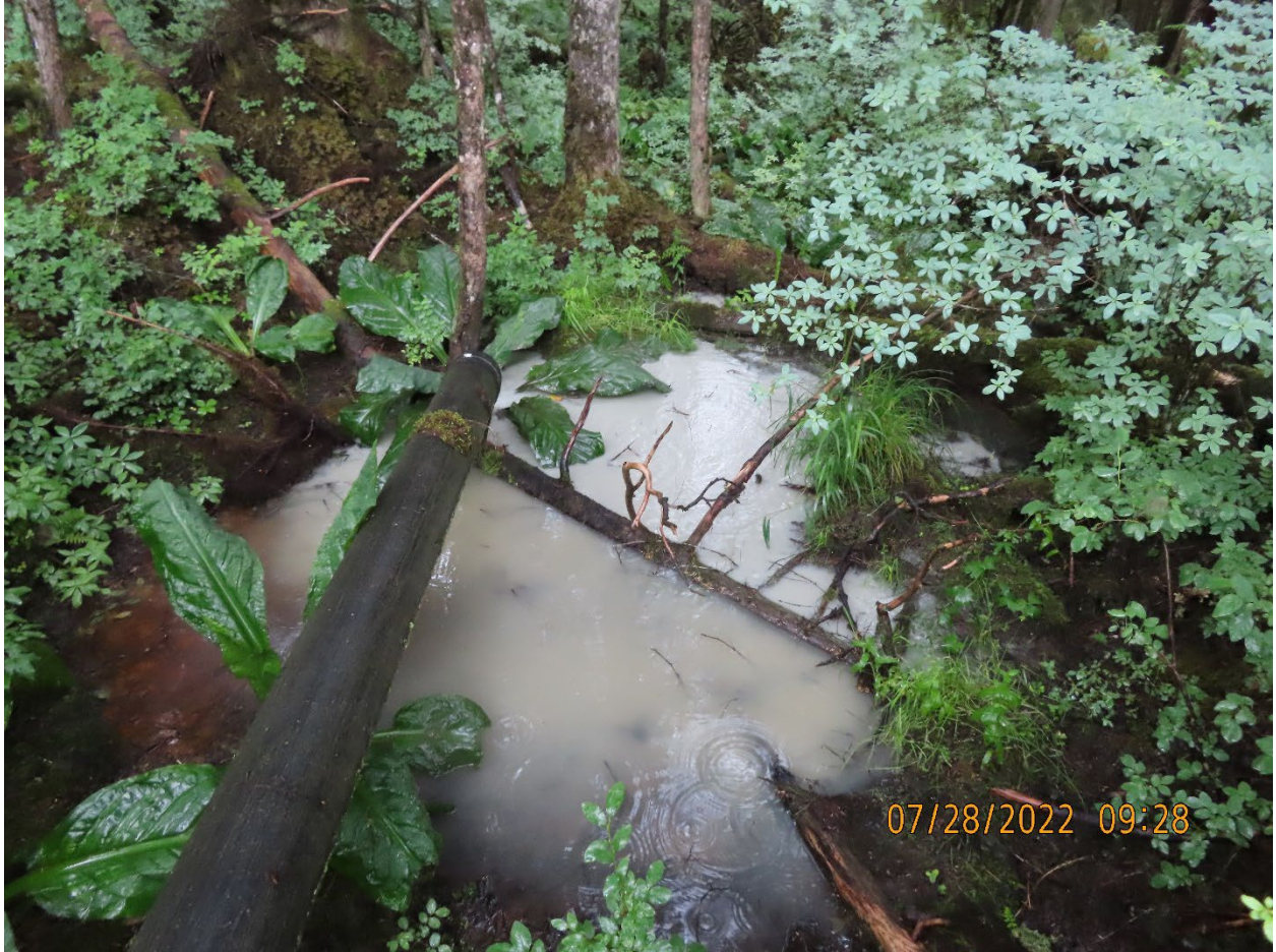
Photo 18. Discharge point of the B-Road Stormwater BMP located uphill from the Zinc Creek Bridge.
