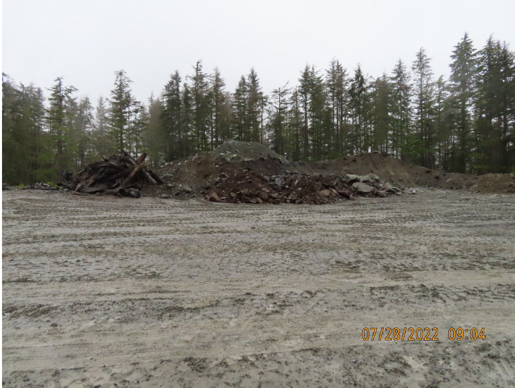
Photo 11. Site E, debris and fill stockpiled from the recently completed slope stabilization work at 5.6-mile B-Road.
