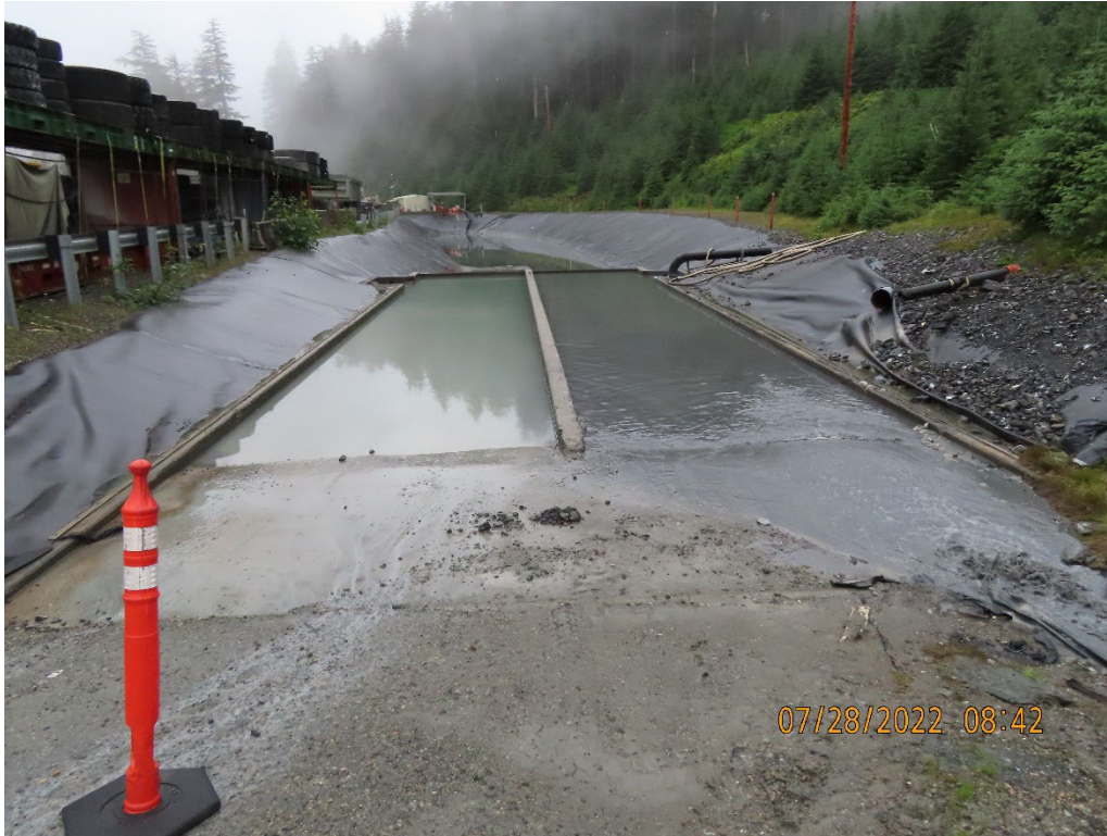
Photo 5. Pond 23 showing substantial surge capacity.
