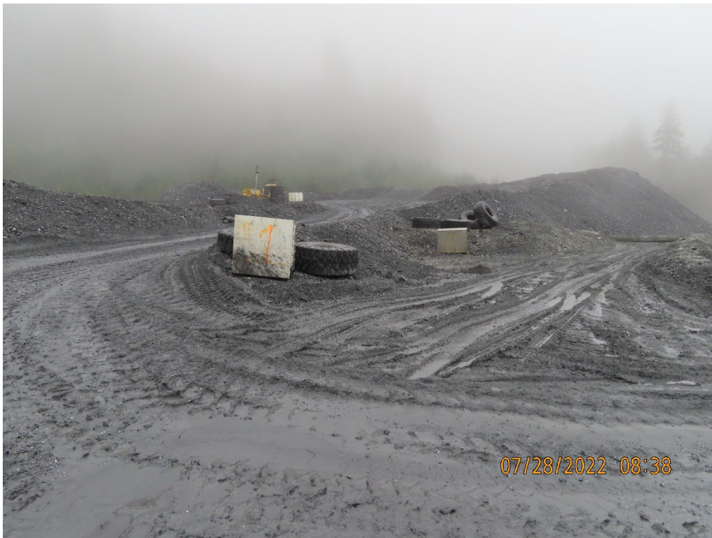
Photo 4. Site 23 active waste rock placement area.
