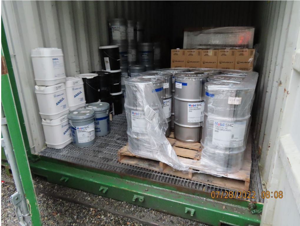
Photo 3. Chemicals stored in appropriate secondary containment at the 920 warehouse.
