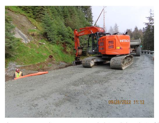
Photo 4. Contractors making emergency repairs to the drainage ditches at the site of the 5.6 mile Broad landslide.
