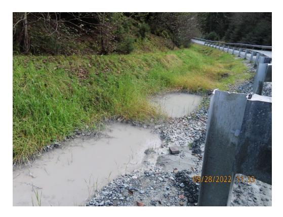
Photo 12. Small sumps above the Gnome Ponds that require sediment removal.
