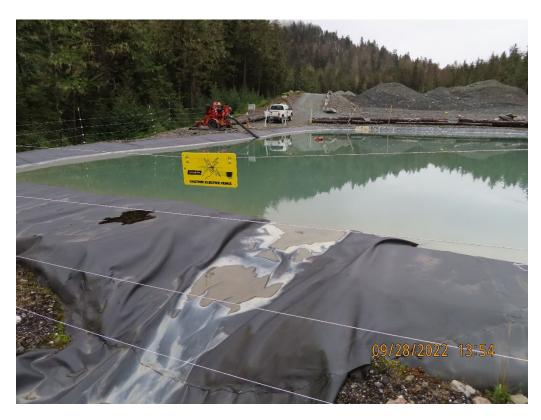
Photo 6. Site E stormwater pond. HGCMC planned to pump water out of the pond.
