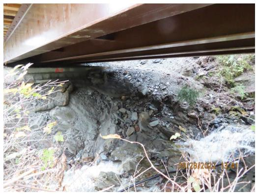
Photo 8. Falls Creek Bridge downhill side abutment BMPs in disrepair.
