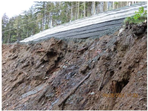
Photo 2. The head scarp of the 5.6 mile B-road landslide undercutting the roadway.
