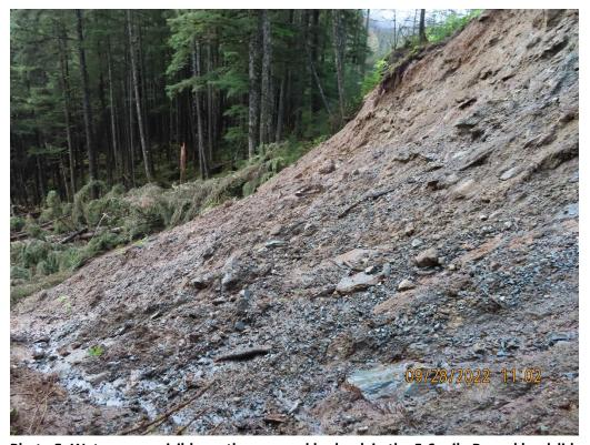
Photo 5. Water seeps visible on the exposed bedrock in the 5.6 mile B-road landslide.
