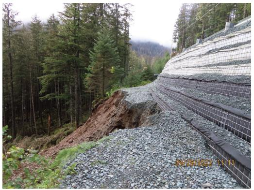
Photo 3. The head scarp of the 5.6 mile B-road landslide undercutting the roadway.
