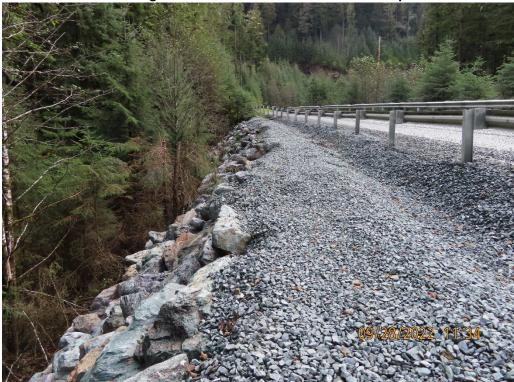
Photo 9. Roadside repairs were completed at the 3.2 mile of the B-Road where a slope failure occurred during the December 2020 storm event.
