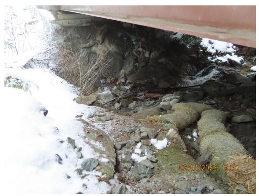
Photo 9. Falls Creek Bridge abutment BMP's.
