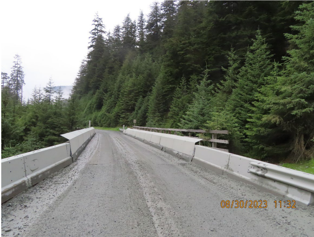
Photo 5. 7.4 B-Road Bridge (Killer Creek Bridge).
