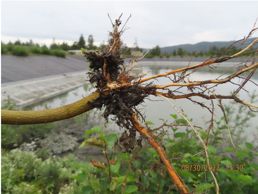
Photo 12. A pulled alder from the soil on top of the Pond 7 liner.
