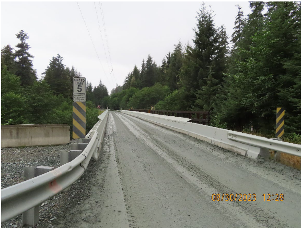
Photo 8. 3.0 B-Road Bridge (Zinc Creek Bridge).
