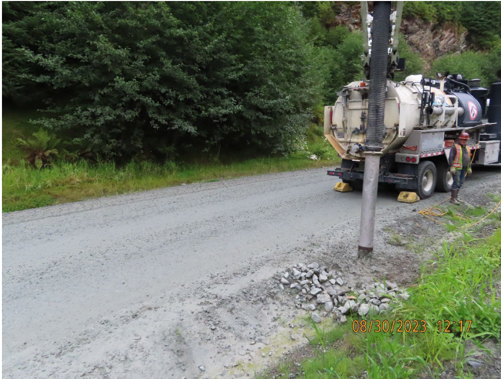
Photo 1. Surface Operations personnel cleaning sumps at the 3.3 Mile B Road.
