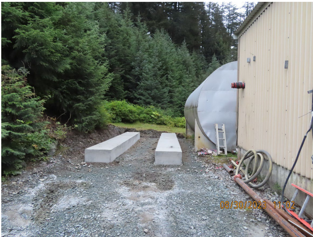
Photo 3. The foundation blocks for the active carbon filtration system.
