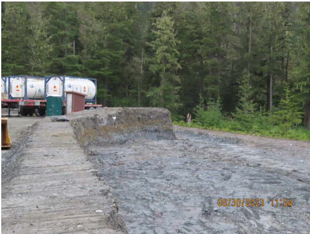
Photo 6. Waste Site E (4.7 mile B-road).
