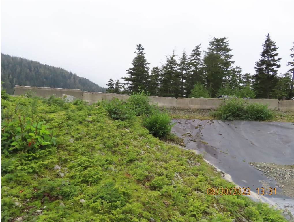
Photo 11. The vegetation is seen growing around the perimeter of Pond 7, has a shallow root system, and is not growing through the liner.
