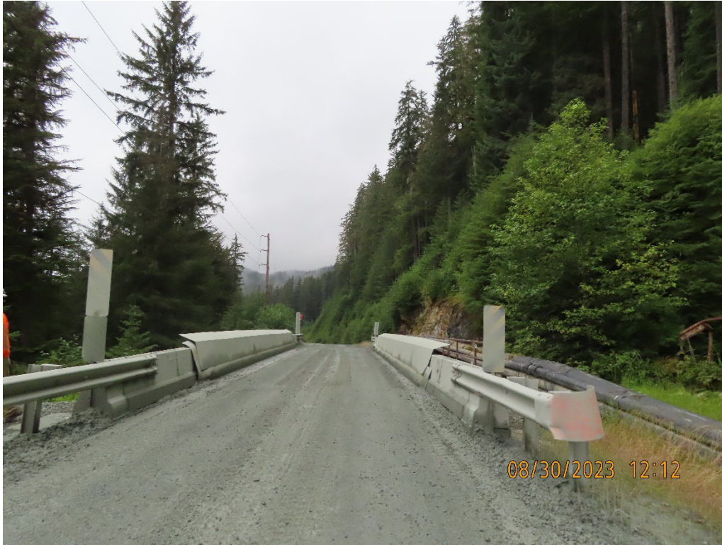
Photo 7. 3.4 B-Road Bridge (Falls Creek Bridge).
