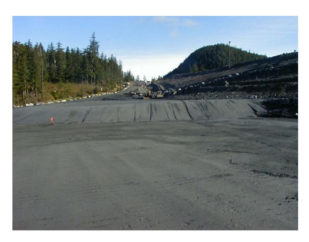
Figure 2.36 Photograph of Compacted West Buttress Tailings
