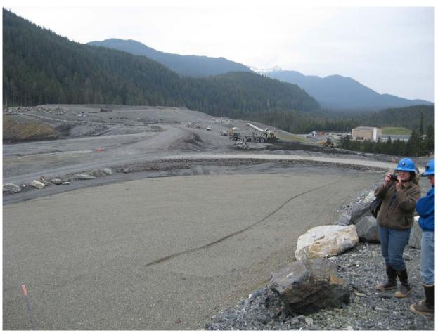
Tailings site; active placement, spreading and rolling under way.
