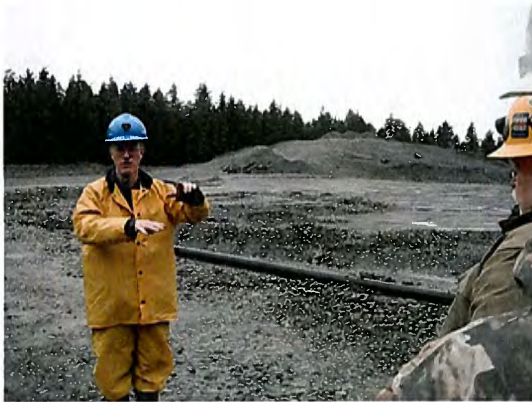
Site E: Approximately 85,000 cy removed
