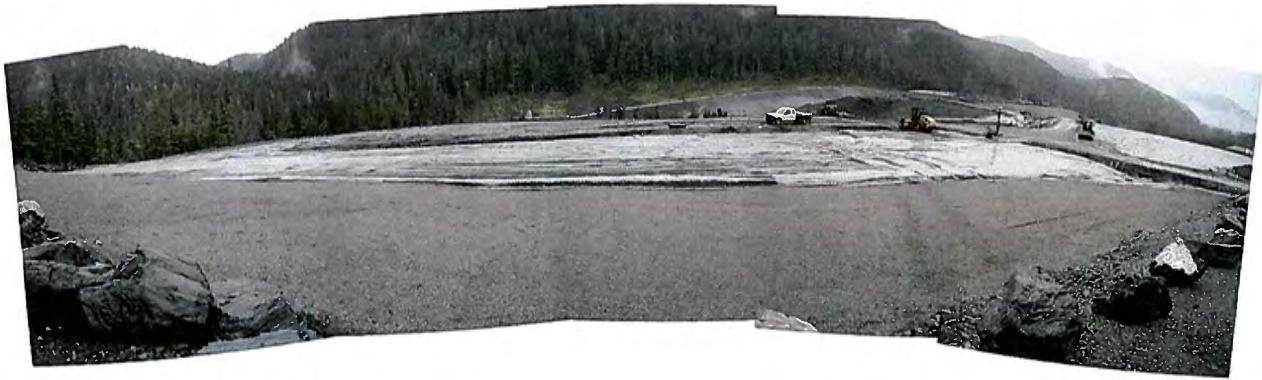
Tailings Disposal Facility: Northwest Expansion area- active placement taking place
