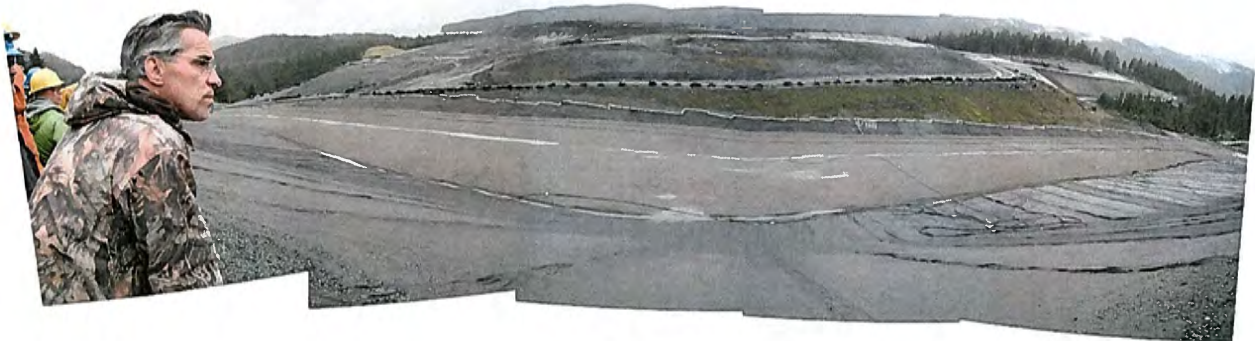
Tailings Disposal Facility: East Ridge Expansion Area
