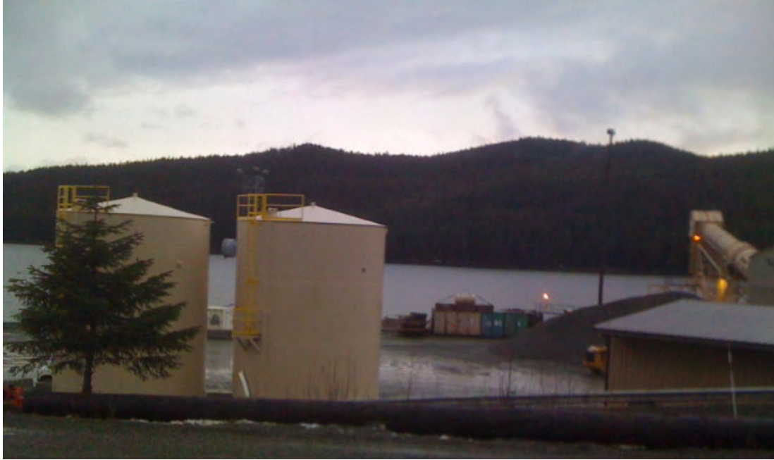
PHOTO 1. Hawk Inlet Storm Water Collection Tanks; Fall, 2010
