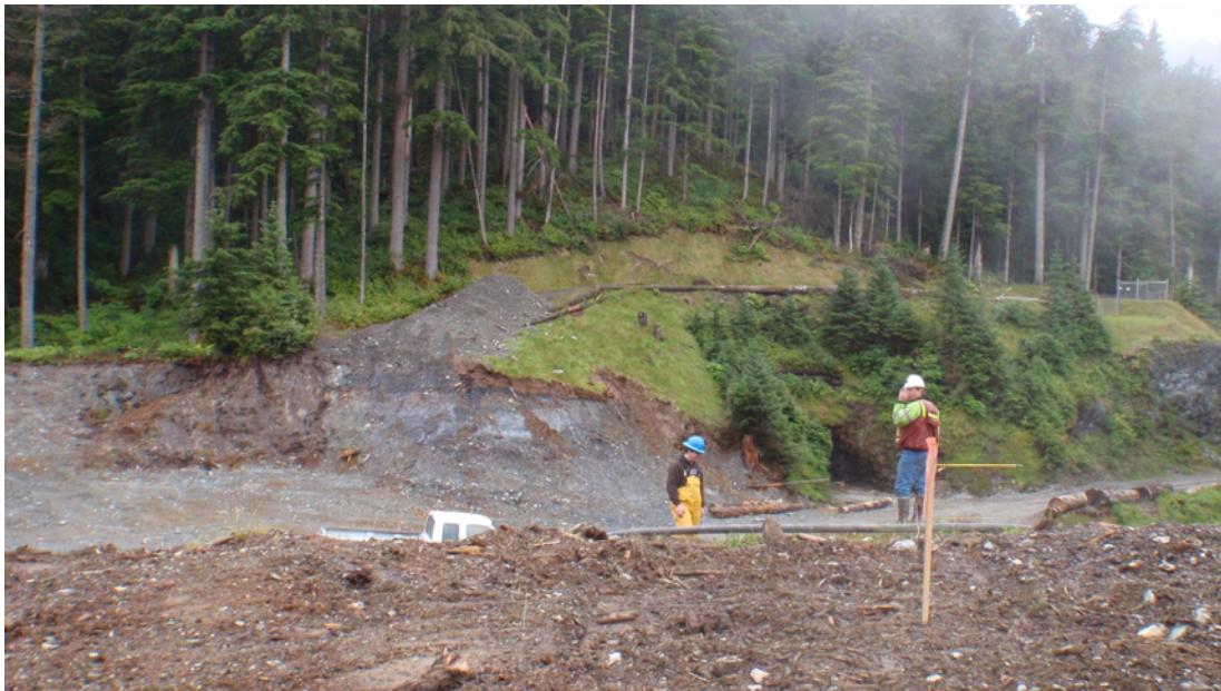
PHOTO 4. Site 1350 Removal Area Near Portal; August, 2010
