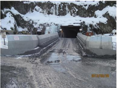
Photo 7. An upcoming drainage improvement project will eliminate ponding around the Greens Creek bridge.
