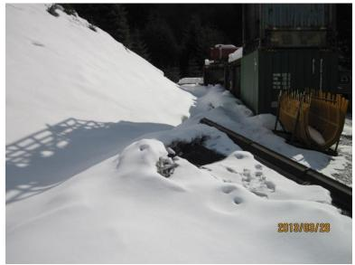
Photo 9. Poor placement of snow push pile adjacent to drainage at the warehouse.
