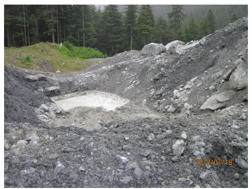
Photo 7. A temporary basin constructed at Site 23 to collect runoff from concrete truck washouts.
