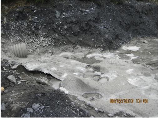
Photo 9. Concrete truck washout pit at Site 23.
