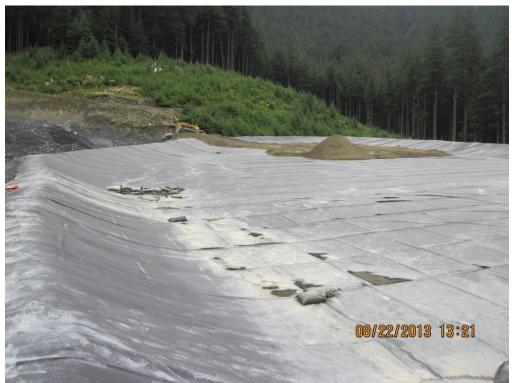
Photo 8. The new liner has been installed at Site 23.
