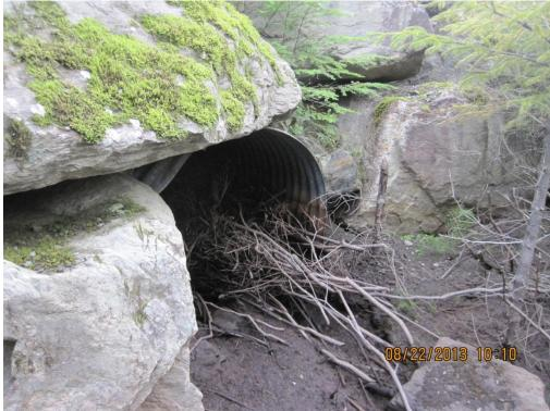
Photo 1. The culvert at A Road milepost 2.2 was clogged with debris.
