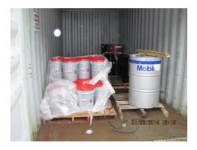
Photo 08. Petroleum products not in secondary containment.
