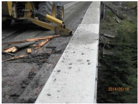
Photo 07. Sediment on top of the splash guard indicates that it should be taller in order to prevent sediment from getting splashed into the stream.
