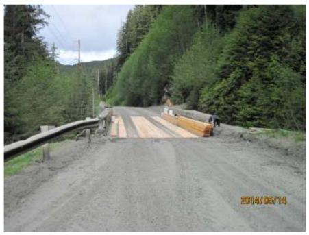
Photo 04. The blanking on this bridge had been replaced just before we drove by.
