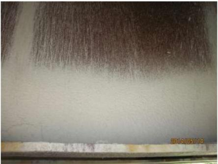
Photo 08. The mud on this girder has fallen through the cracks in the bridge planking. Some of the mud will fall directly into the stream.
