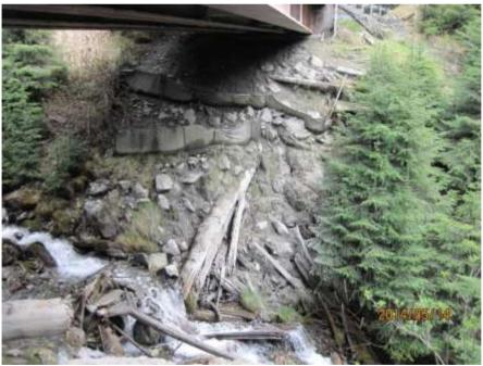
Photo 06. Silt Fences are capturing some of the sediment underneath the bridge, but there is a lot of sediment beyond the lowest silt fence that will get washed into the creek when it rains.
