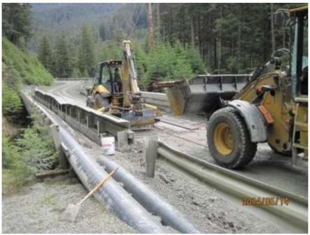
Photo 05. The planking of the bridge at mile 7.4 on the B Road was being removed by an excavator, and hauled away by a loader.
