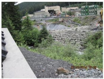
Photo 06. Repaired riprap along outer berm of Pond A.
