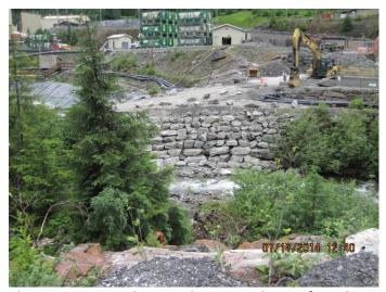
Photo 07. Repaired riprap along outer berm of Pond A.
