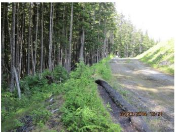
Photo 19. Sediment barrier disturbed by bear activity at Site E.
