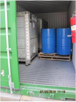
Photo 09. Reinforced totes stored with insufficient secondary containment.
