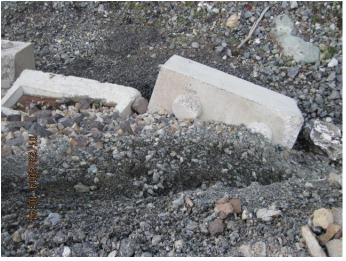
Photo 04. Retaining wall knocked over.
