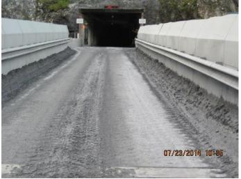
Photo 01. Accumulated sediment on the 920 bridge.
