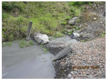
Photo 08. Settling basin full of sediment.
