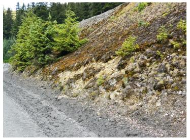
Figure 10 Slope next to the Haul Road showing signs of movement.
