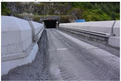
Figure 3 Sediment on the bridge leading to/from the portal.
