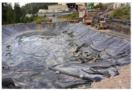
during the inspection. The liner was being removed, and preparations to reline the pond were underway (Figure 13). Water that normally would have flowed to A Pond was being stored in a degrit basin and pumped to Pond 23, then to Pond 7 at the TDF. Soil was being excavated from an area near the mill building after a failed fitting led to a
