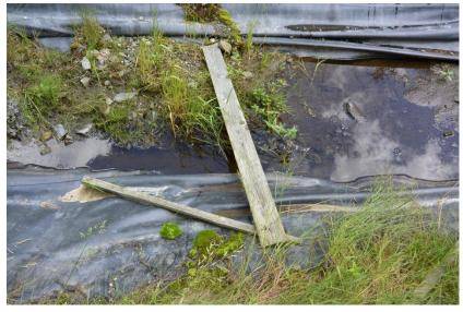
Figure 11 Vegetation and debris in a diversion ditch.
