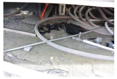
Figure 14 Oil floating on water in secondary containment.
