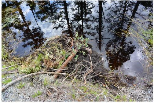
Figure 18 Debris placed at a culvert inlet by beavers.
