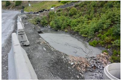
Figure 9 Settling pond full of sediment.
