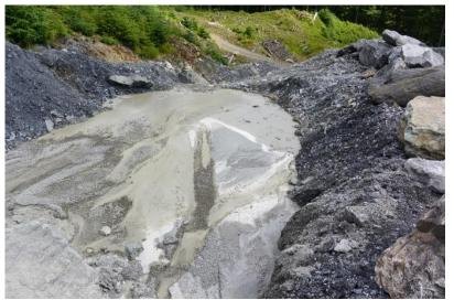
to tell whether the orange stains were due to organic iron bacteria, or acid generation/metals leaching. The in situ settling basins at Site 23 were also full, and not performing as designed (Figure 16). The team walked along the drainage path that carries water from Site 23 down to Pond 23, and then walked across the B Road to the pipe outlet that delivers water to D Pond. D Pond is overgrown with vegetation. Much of the vegetation had been pressed flat,
