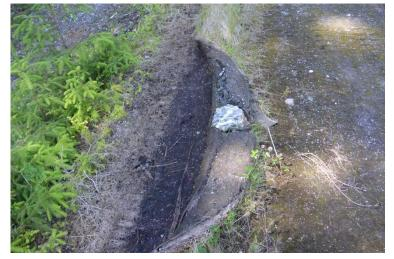
Figure 17 Permeable mesh pulled back by bears.
