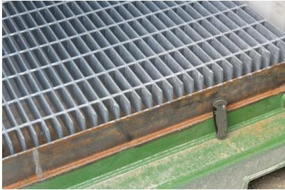
Figure 2 Added freeboard to the integrated secondary containment.
