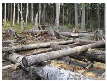
Photo 08. Killer 23, pad partly constructed of cut trees. Dimensioned lumber removed.
