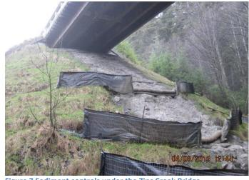
Figure 7 Sediment controls under the Zinc Creek Bridge
