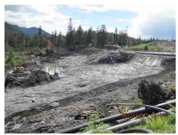
Photo 14. Excavation of soil at southern end of TDF.
