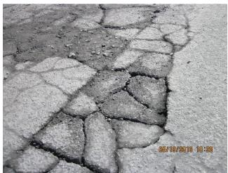
Photo 9. Zoomed in image of the cracks in the 920 concrete overlay.
