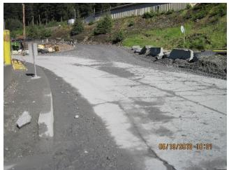
Photo 10. Cracks in the 920 concrete overlay.
