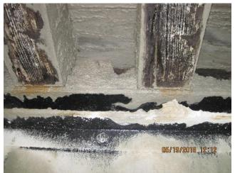
Photo 13. Sediments from B-road permeating through the wood planks.
