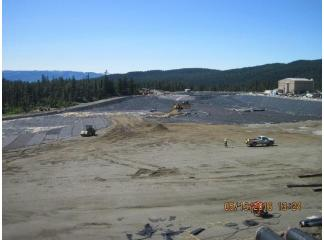
Photo 22. HDPE liner installation at the TDF expansion site.
