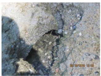
Photo 14. A culvert near Falls Creek Bridge needs mucking.
