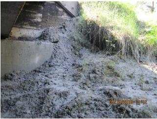
Photo 12. Sediments from B-road accumulating below the bridge.
