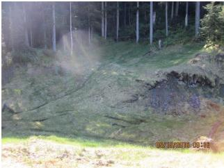
Photo 3. 1350 re-hydroseeding for exposed rock pile.
