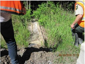
Photo 15. Collapsible drainpipe south of the Falls Creek Bridge.
