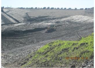
Photo 27. HGCMC personnel excavating tailings to improve contact water drainage into Pond 9.
