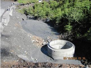
Photo 6. Rock check dam and sump across from DB-01 need mucking.
