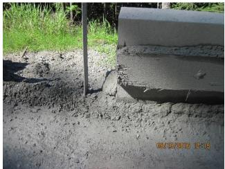
Photo 11. Sediment buildup at the edge of Falls Creek Bridge.
