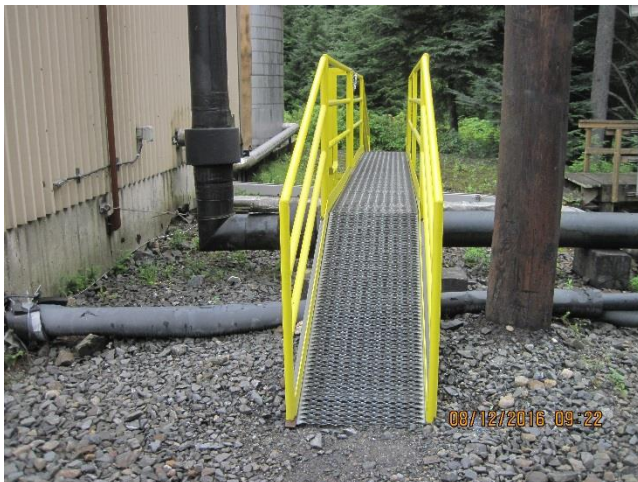
Photo 6. 920 Pump house safety improvement.
