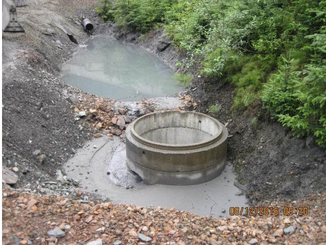
Photo 4. 920 sump across from DB-01.
