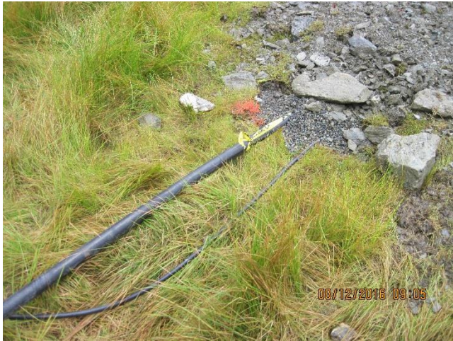
Photo 2. Pipeline for the 1350 caisson to the 1350 adit.
