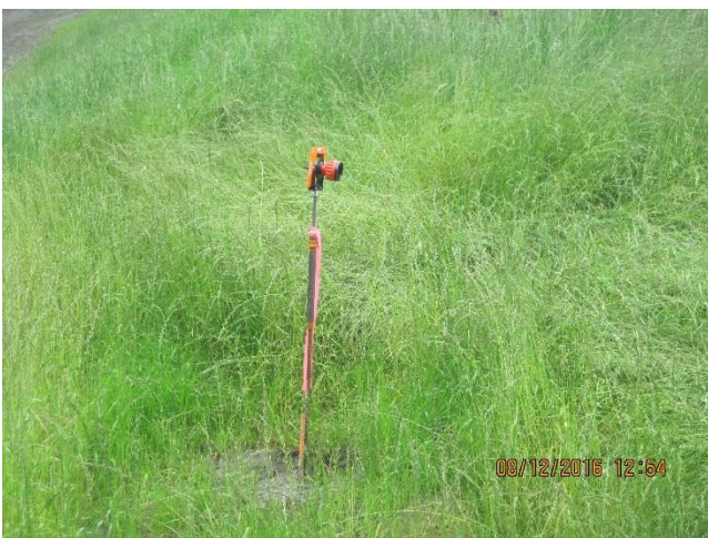
Photo 27. A prism monitoring system for monitoring slope movement.
