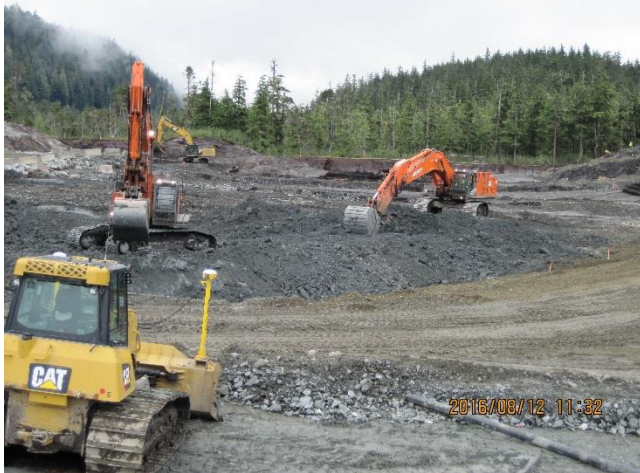
Photo 22. Gray/blue clay excavated from Pond 10 is stockpiled at the Sand Pit.
