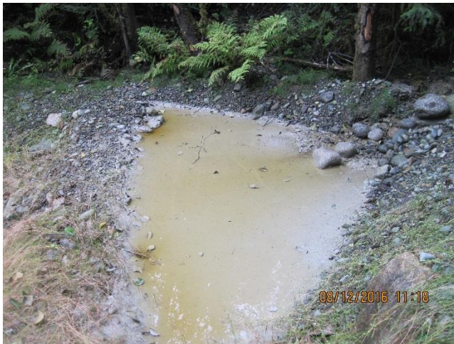
Photo 17. Settling sump near capacity.
