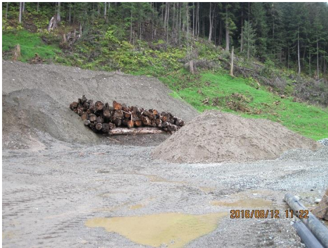
Photo 23. 0.9 mile sand stockpiles.
