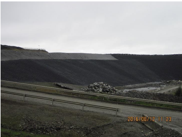
Photo 21. Class-1 waste rock deposited on the outer slopes.
