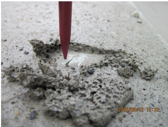
Photo 11. Sediment accumulation on the Killer Creek bridge's rails.
