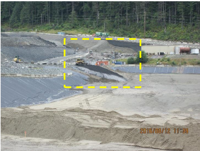
Photo 20. Highlighted within the dashed lines, tailings are now being deposited at the TDF expansion.
