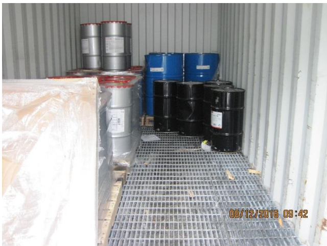
Photo 9. 920 warehouse storage container with secondary containment.
