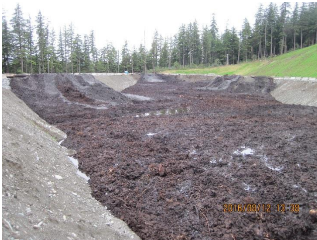
Photo 29. Organic material stockpiled. Approximately 1/5 of the pit is full of organics.
