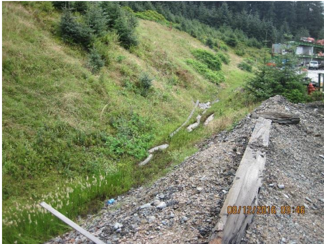
Photo 7. Water diversion ditch behind the 920 ore pad and warehouse.
