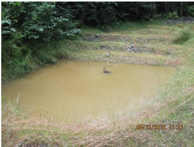
Photo 18. Some sediment is working its way through the sumps and rock check dams.
