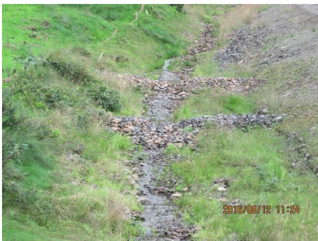
Photo 24. Rock check dam.
