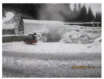
Photo 3. DB-01 with snow mixed with sediments from plowing. The sediments are captured and the melt water drains into 920 Pond-A.
