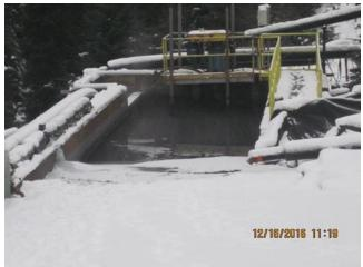
Photo 4. DB-02 sediments are captured and the water drains into 920 Pond-A.
