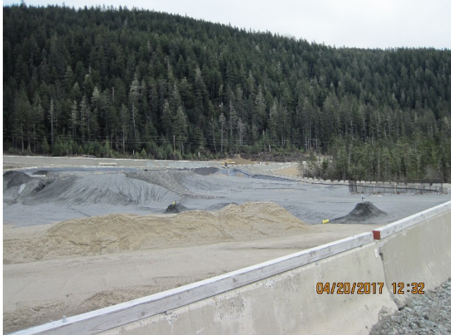
Photo 12. Southern expansion TDF (S3P1).
