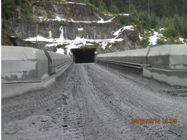
Photo 01. 920 Portal and Bridge.
