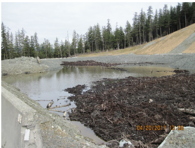
Photo 14. A-road Sand pit.
