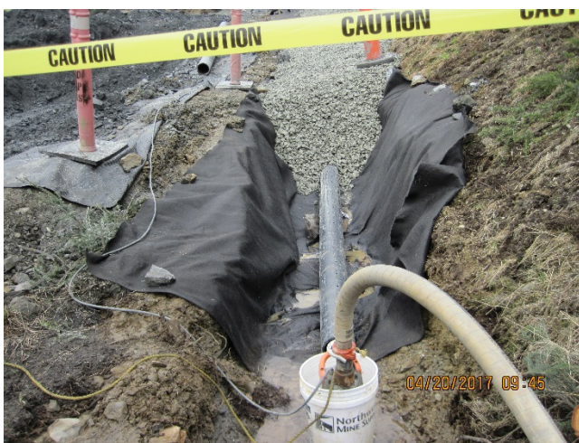
Photo 05. Diversion ditch upslope of the Ore Pad.
