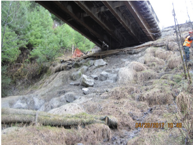
Photo 10. 3.0-mile Zinc Creek Bridge
