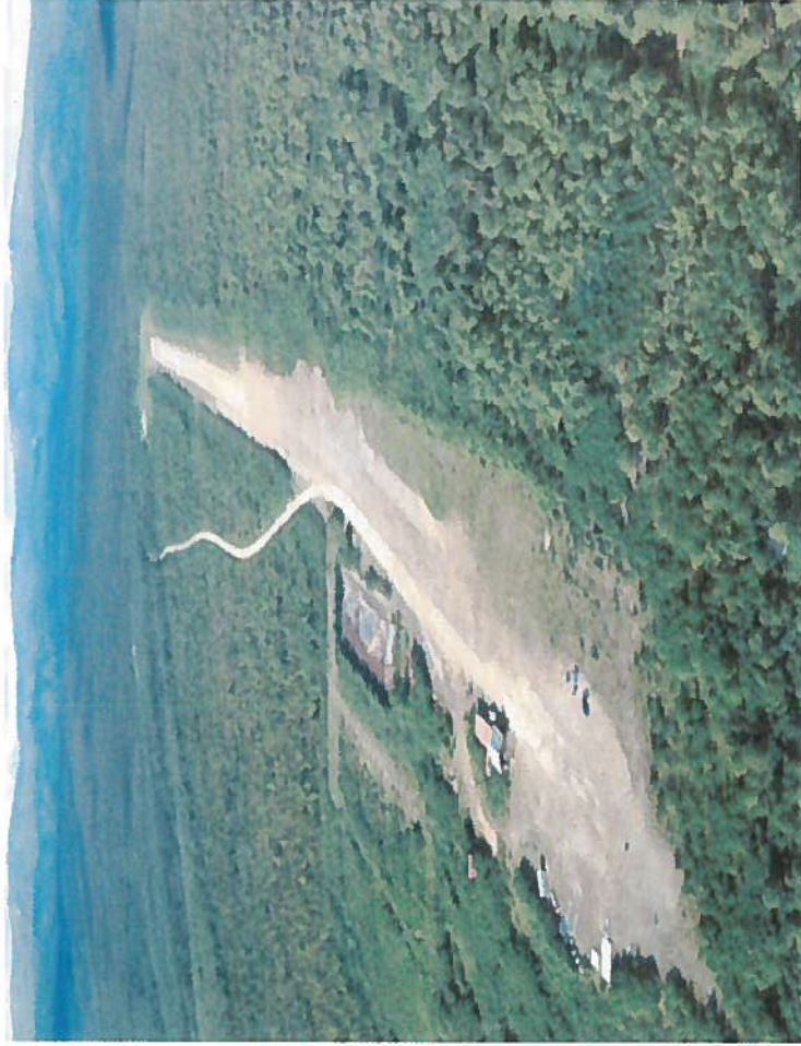
4,400 Foot Airstrip with fuel storage Heavy equipment on site for loading DC-6/C-130 Capable
