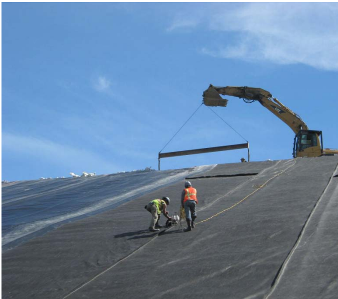
PHOTO 3. STITCHING GEOTEXTILE ON THE DAM FACE
