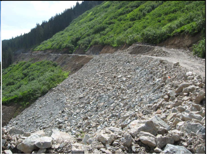
PHOTO 10. PIPELINE – SNOWSLIDE GULCH AREA
