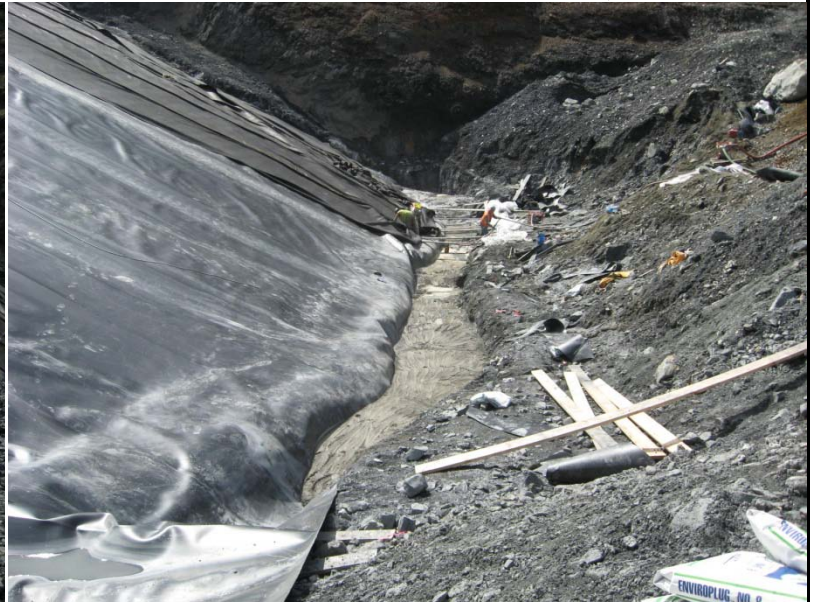
PHOTO 2. LINER AND GROUT TRENCH
