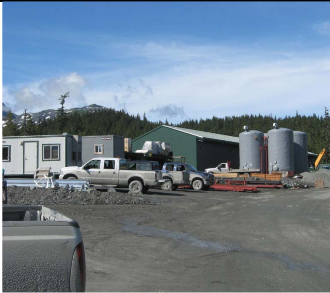
PHOTO 9. TTF WATER TREATMENT PLANT
