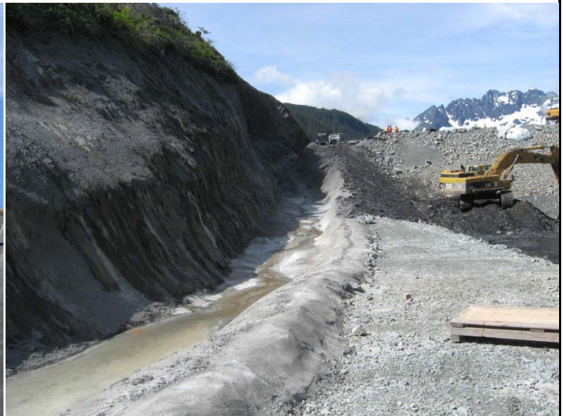
PHOTO 4. CONCRETE LINED SPILLWAY
