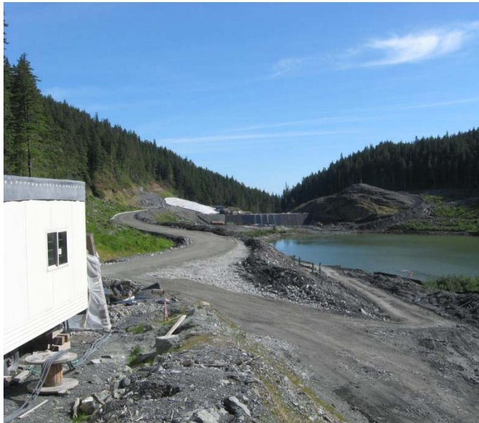
PHOTO 11. GENERAL VIEW OF TTF AND DAM
