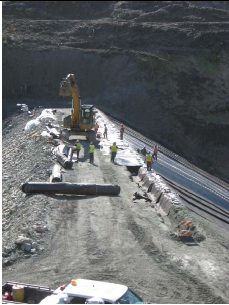
PHOTO 5. ANCHOR TRENCH AT TOP OF DAM
