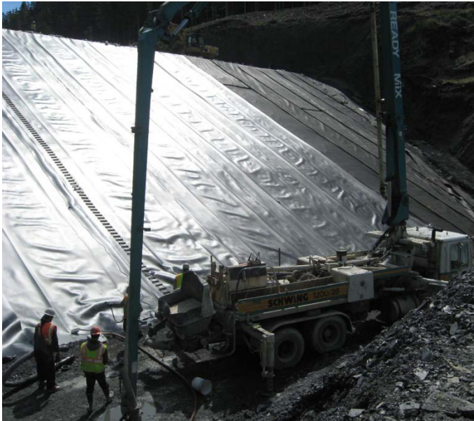
PHOTO 1. DAM GEOTEXTILE & GROUT PUMP
