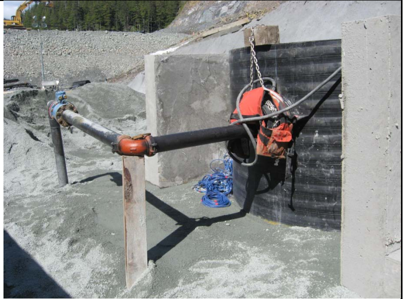
PHOTO 6. FLOW METER AT DAM SEEPAGE SUMP
