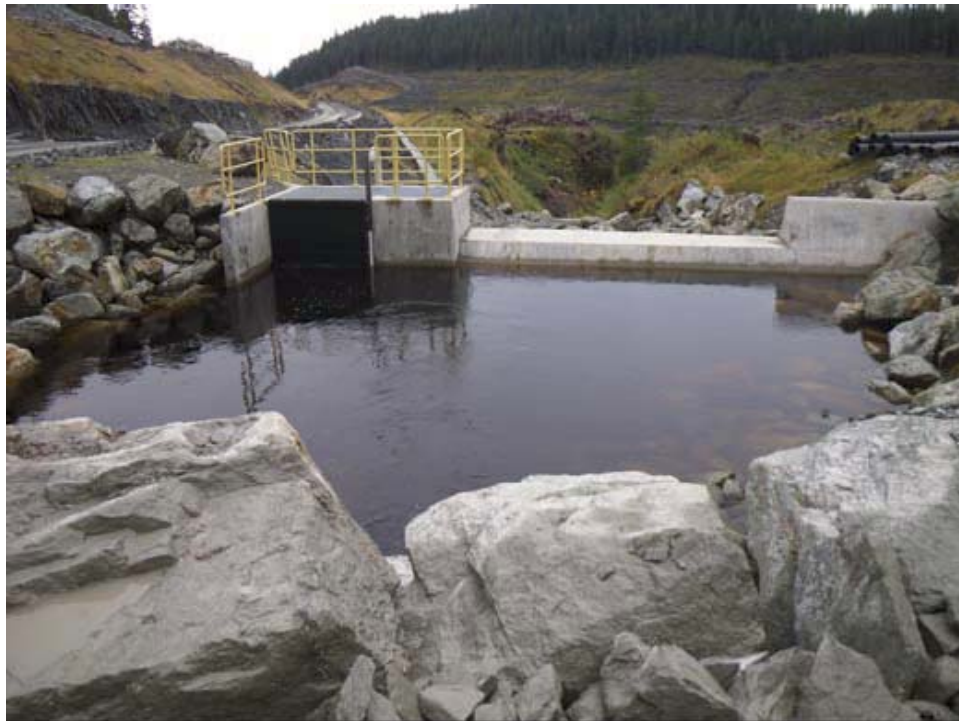
Figure 3: Diversion dam; water enters a 36 inch pipe underneath yellow railing.
