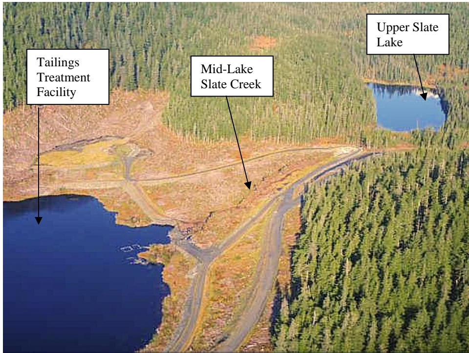
Figure 2: Mid-Lake Slate Creek with water restored to the channel.
