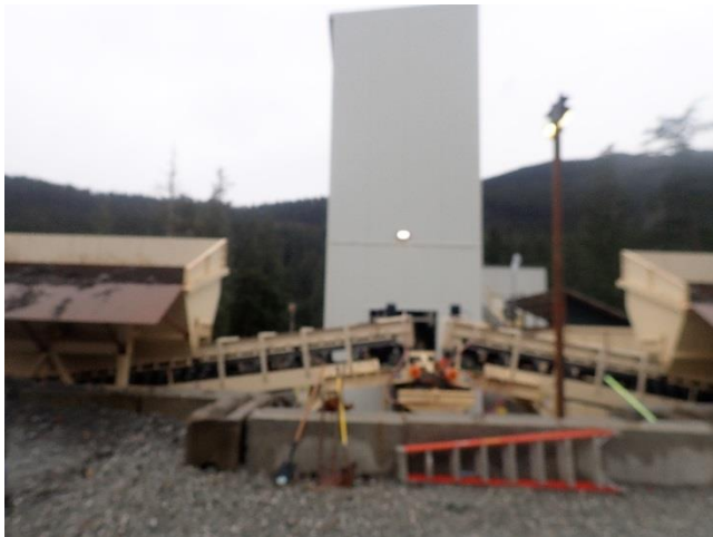
Photo 19. The Pug plant located at Pit 4.
