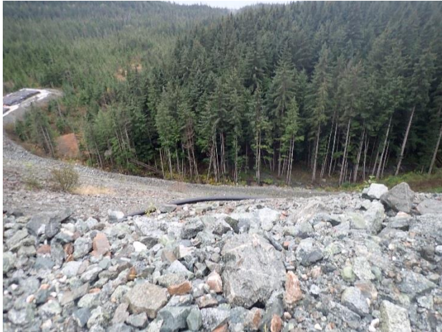
Photo 1. The Comet development pile.
