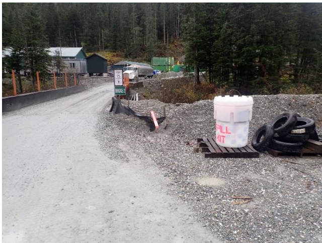
Photo 12. A portable spill kit staged near Bridge 2.
