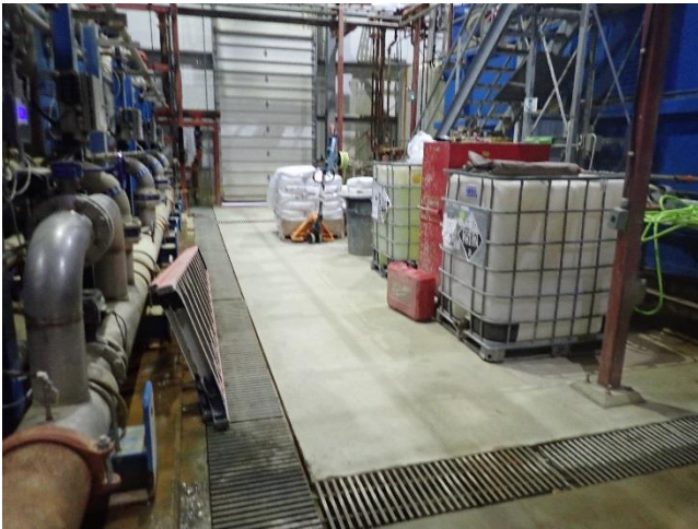
Photo 5. Inside the CWTP.
