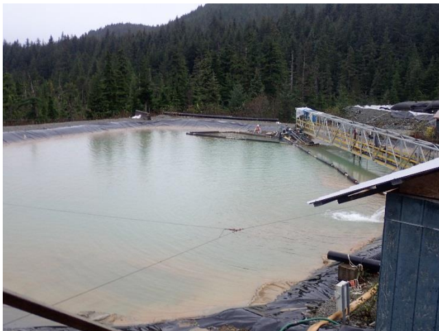
Photo 3. The CWTP's Pond 2.
