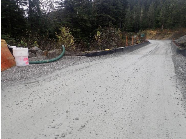
Photo 13. A portable spill kit staged near Bridge 1.
